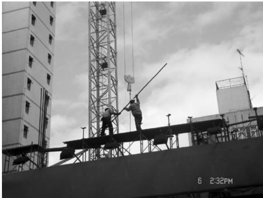
Figure 2.10 - Working at Height for Steel Fixing
