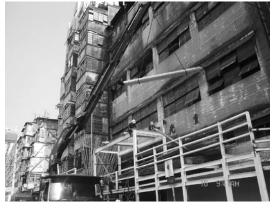
Figure 2.11 - Working at Height for Hoarding Installation
